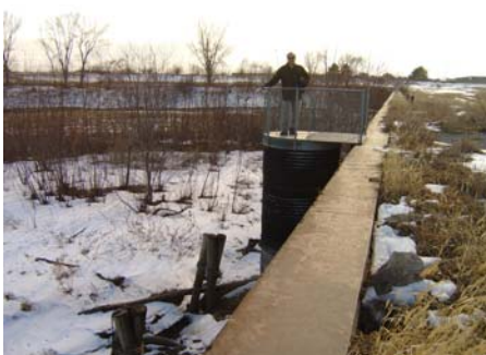
Abandoned Missouri River Barge Canal pump location
