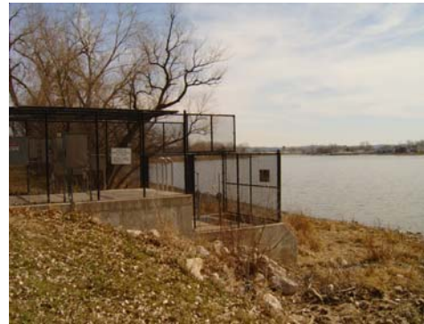
North Flood Control Lift Station
