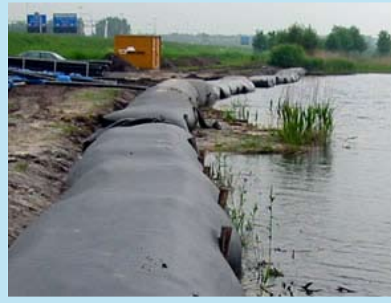
Geotube example (construction)
